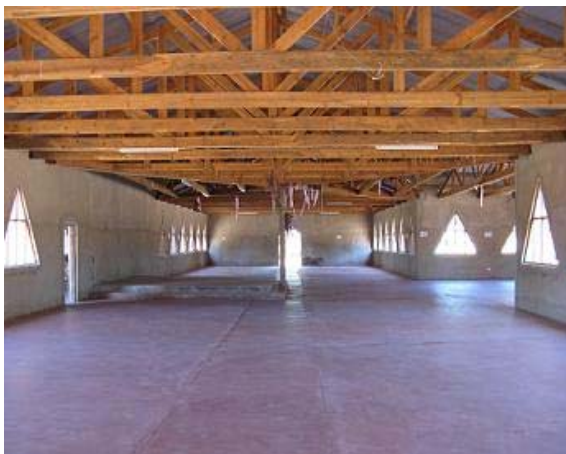
Presbyterian Church at Kalikumbi before installing pews.
